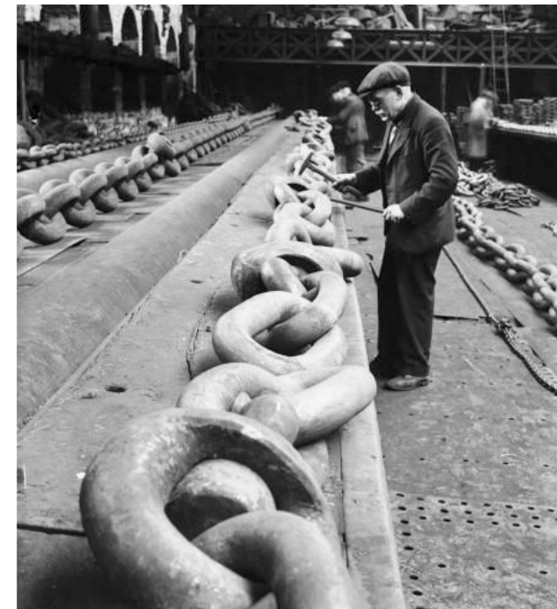
March 1936, a worker testing the links of a giant chain in a chain works in Pontypridd, South Wales (photo by Fox Photos / Getty Images)
