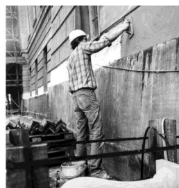
Repairs on the Humboldt main building Source: Humboldt-Universität / Archive
